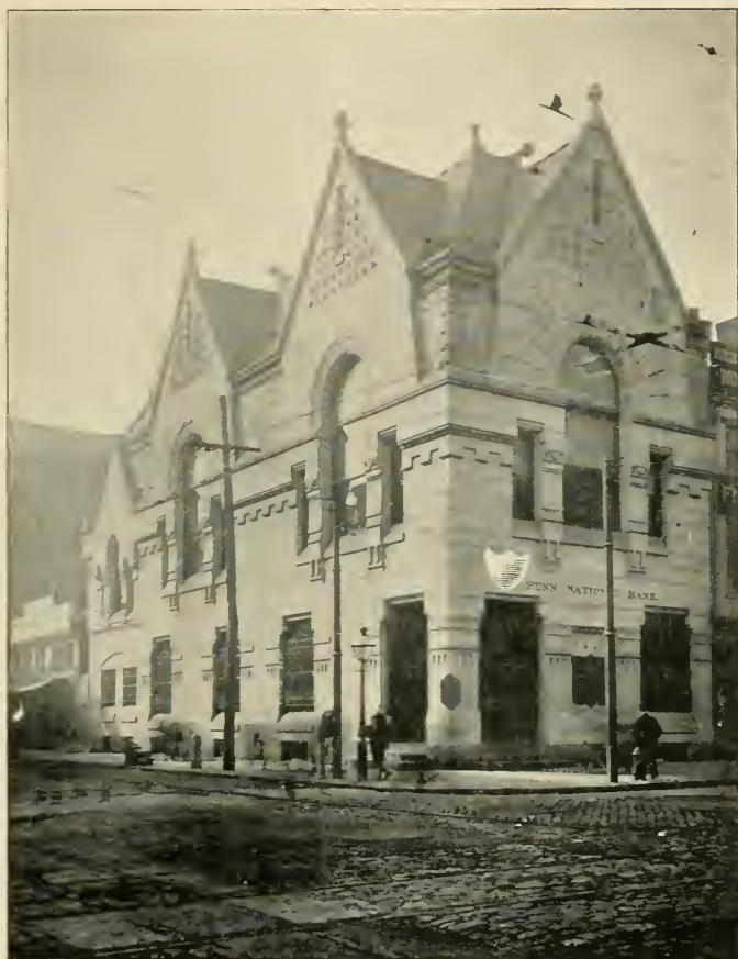
CORRECT POSITION OF MEMORIAL SHIELD ON PENN NATIONAL BANK BUILDING.
